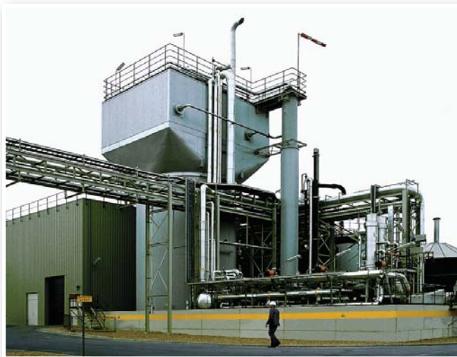
Budel zinc refinery - hydrogen gas lift loop reactor for sulphate reduction and zinc recovery.
